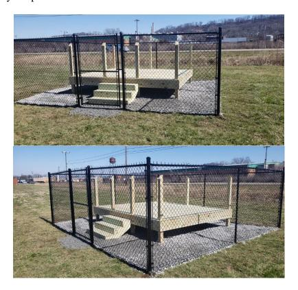
Preliminary measurements were made at the site to ensure that the sampler is at least 10 meters from any trees and that the sampler has 270° unobstructed fetch for wind flow, and indicate that the sampler meets the siting criteria in 40 CFR 58, Appendix E. The information below shows the site details for the new Rossville-Williams St. monitoring station.
